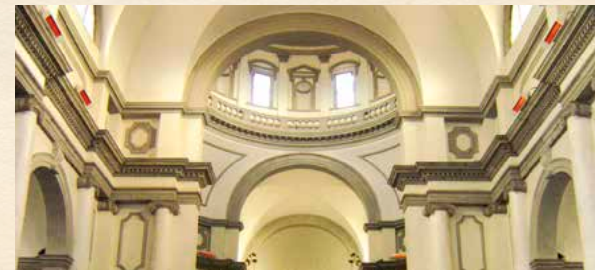
SUNRAD radiant heating system in the Cathedral of Castelfranco Veneto - Treviso - Italy
